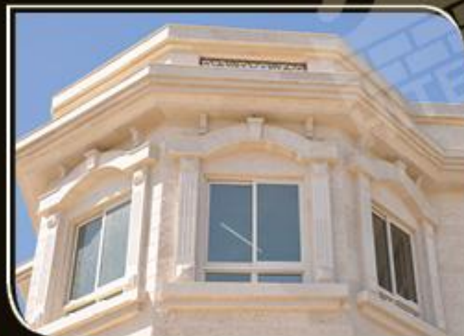
Palastinian Stone White polish & Mufager for flat area & Palastinian White polish for Decorations. (Dubai - Al Tawar)
