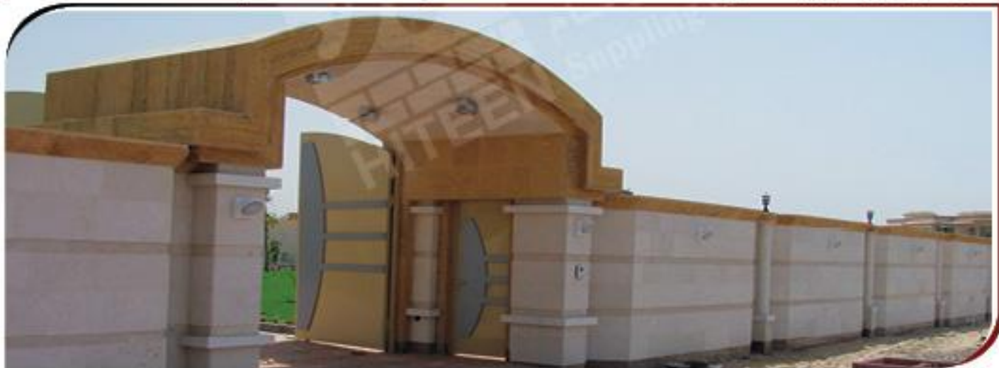
Saudi stone White Bush hummer & polish White for flat Area & Saudi yellow Stone for decorations. (Dubai - Nad Al Shiba)
